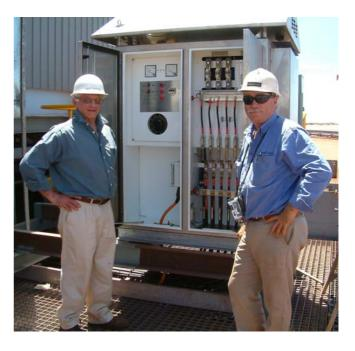
Convection air cooled TR. Marine grade aluminium cubicle.
