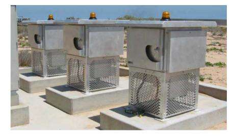
Convection air cooled TR 3 phase operation
